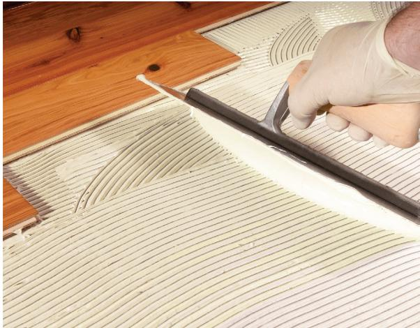
No. 03732). Maximum acceptable floor variation is 3/16" in 10 feet. Areas requiring patching or leveling must be done using a Portland cement-based material (e.g., Bostik UltraFinish™ Pro, Webcrete® 95, Webcrete® 98, SL-100™, SL-150™, SL-175™ or SL-200™).
